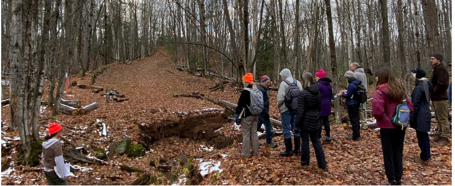
UPLC Staff and community members at Vielmetti-Peters Reserve share ideas for the bridge replacement over Midway Creek.
